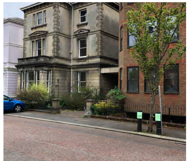
Villas and commercial uses on Clanricarde Gardens
