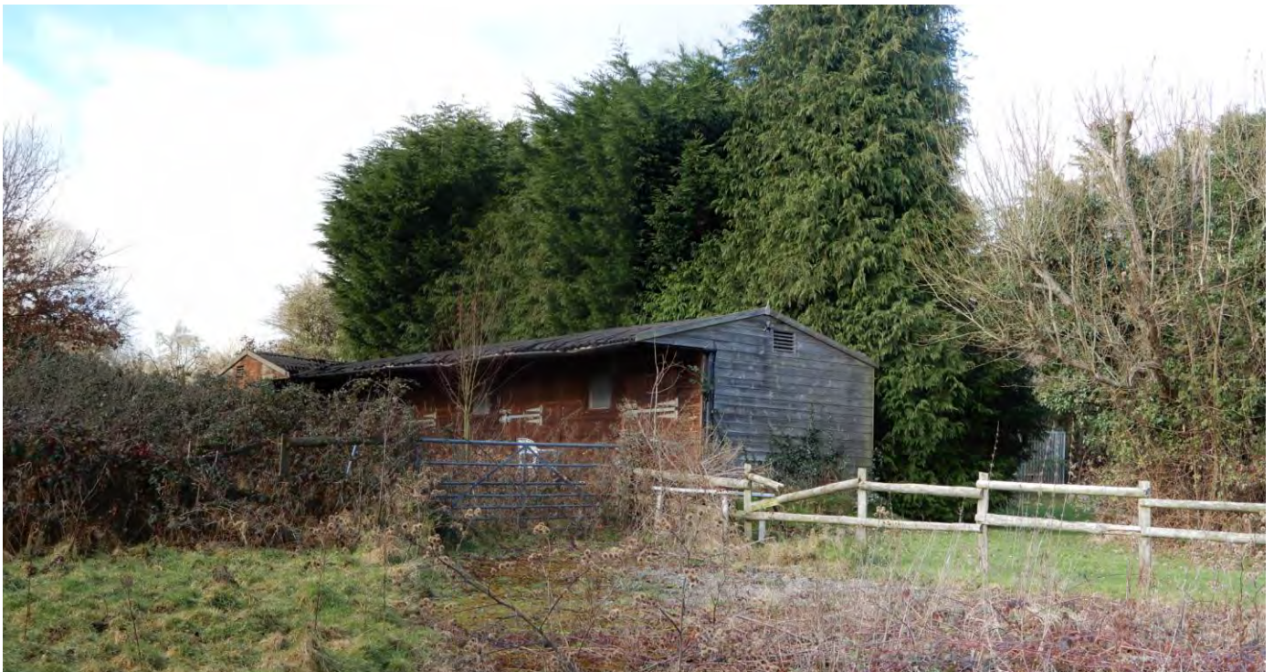
17. View west from the central part of the site, showing the timber stable block with a line of tall conifers behind it. Two images combined, February 2022.
