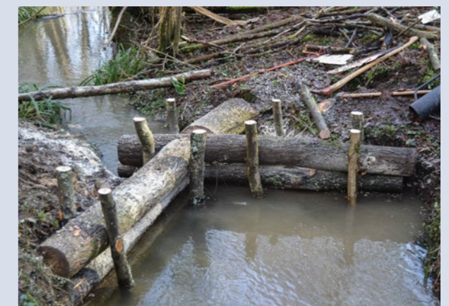
Above: Natural Flood Management measures such as leaky dams reduce and control flood surges in the area.
