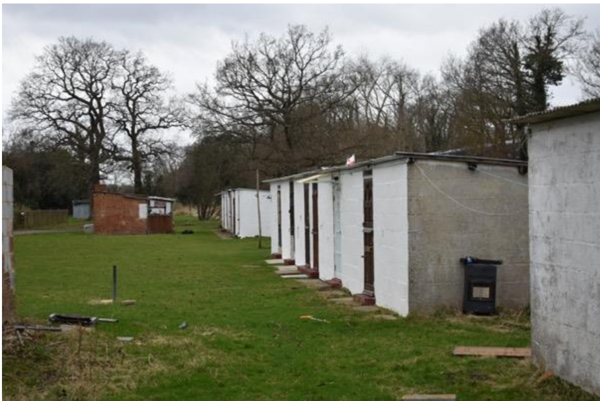
Photograph showing white breeze block Hoppers Huts still in good condition
