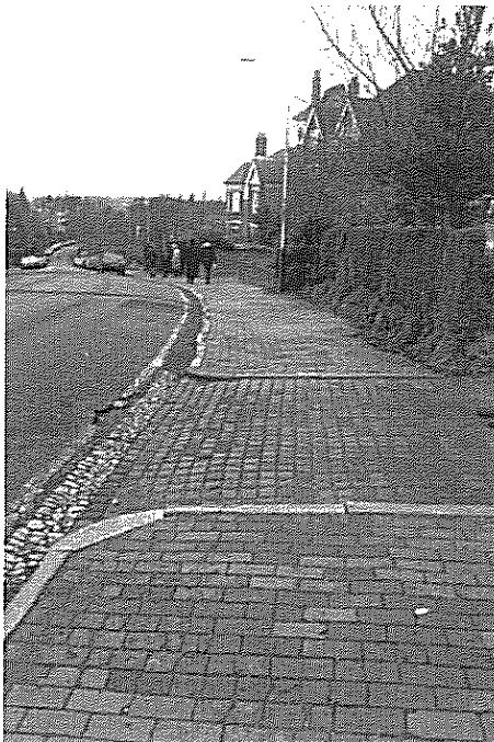
Ground surfaces, Boyne Park
