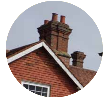
Chimneys and slate roofs
