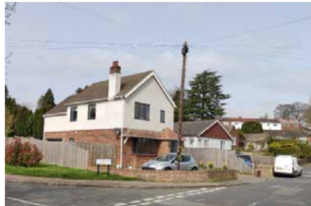
Figure 17: Positive example of corner building.
