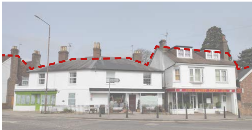
Figure 53: Photos showing a local example of roof variation.
