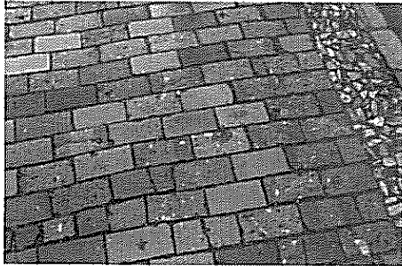
Ragstone spalls and brick paving detail
