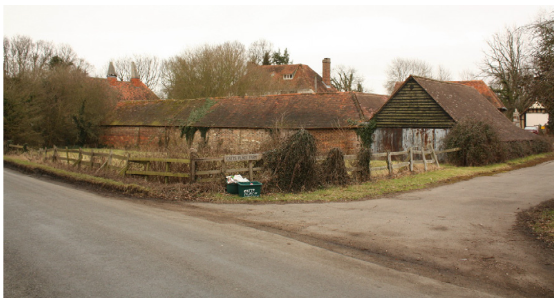
Figure 6 A characteristic larger Wealden farmstead group forming a courtyard with the 17th century farmhouse. The traditional farm buildings include two timber-framed barns, one of which has been partly converted to an oast house, stabling and cattle housing with a mixture of gabled and hipped roofs, framing with weatherboarded walls, brick and clay tiles
