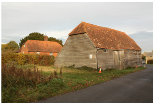
A loose courtyard group with a four bay barn aisled to the rear and with a half hipped roof. The medieval farmhouse stands across the yard from the barn.
