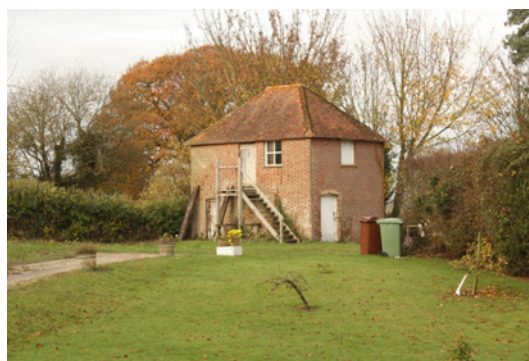
A brick-built stable with a granary above. Granaries in the Weald are typically found above stables or cart sheds or formed part of the barn. Free-standing granaries are rare.
