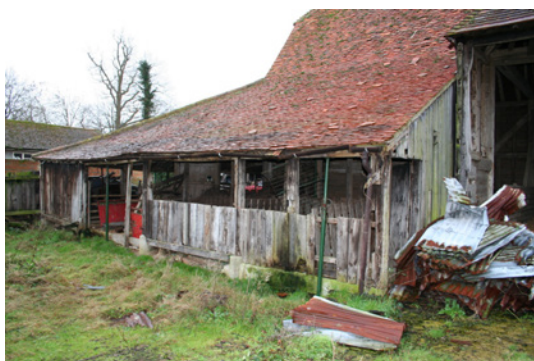
In the 19th century cattle were typically housed in open-fronted shelter sheds which could be attached to the barn or freestanding, often facing into a yard. Open fronted sheds were also used to house tethered cattle.
