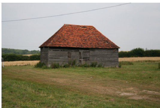
Stables are generally small buildings in the Weald. This single storey timber-framed example has a characteristic hipped roof.
