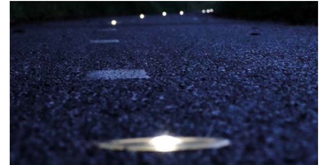
Figure 60: Example of a foot/cycle path which is lit by solar cat's-eye for pedestrian and cyclists, minimising disturbance to nearby properties and natural habitats.
