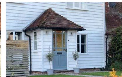
Figure 32: Enclosed porch with a clay tile hipped roof and matching white weatherboard to the house facade
