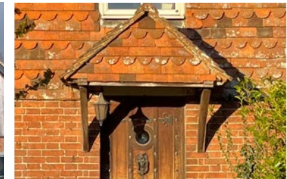
Figure 29: Hipped timber porch with matching clay hung tiles to the house facade
