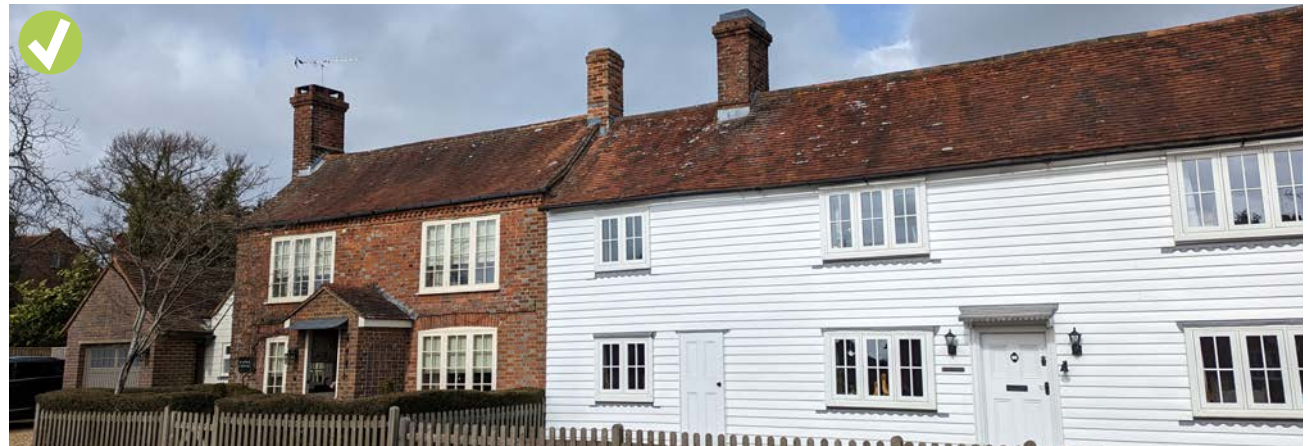
Figure 78: Local example of terraced housing. This typology provides more efficient envelopes compared to semi-detached or detached houses.
