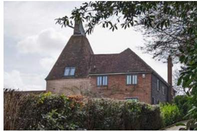
Figure 24: Oast house with hipped roof stowage & square kiln with pyramidal roof
