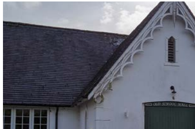
Figure 27: Cross gabled roof with slates & decoration.
