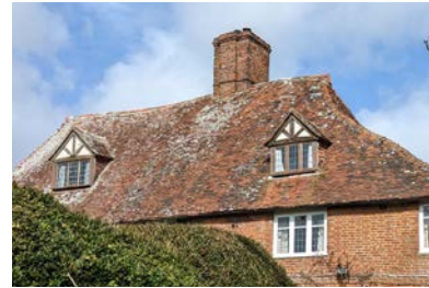
Figure 25: Older roof with kent peg tiles, brick chimney & dormer window
