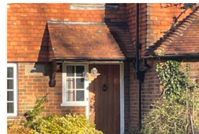
Figure 31: Half-gabled hooded porch with clay tile roof that blends in with red hungtiles used on the property facade
