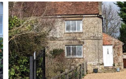
Figure 38: Sandstone & red brick side extension
