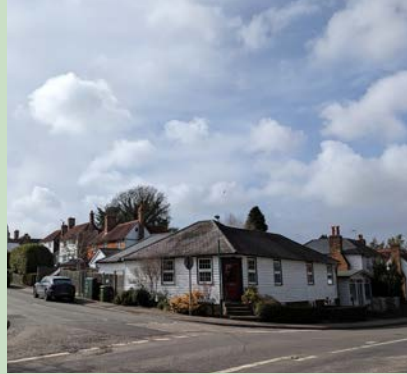
Figure 06: Old Post Office set in the corner of the main road and opposite to the village green acts as a landmark and focal point for the village.
