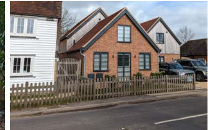
Figure 44: Low height timber fencing (with gaps)
