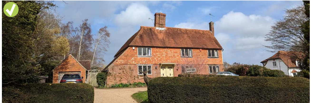
Figure 77: Local example of a south facing property (approx. 30 degrees) that maximises the solar gain, whilst plantation to the north offers protection from cold northerly winds, Queen Street.
