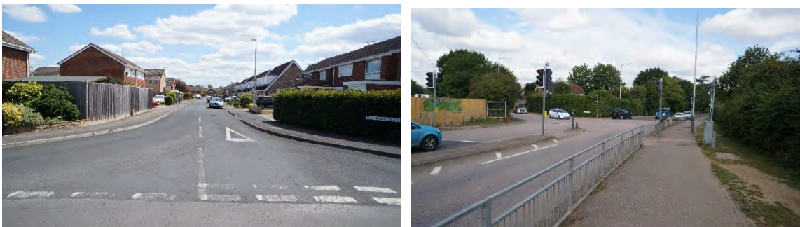
Figure 4-20: Example of wide-splayed junction at Warrington Road (left) and precedent image of a continuous footway treatment on right (Willow Street, Hackney)
