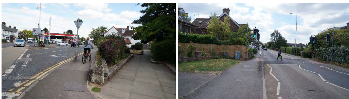
Figure 4-27: Photos of Maidstone Road/Commercial Road Junction
