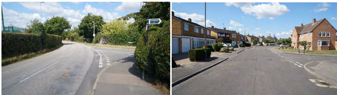
Figure 4-21: Green Lane and Warrington Road are two of many side-entry junctions in the town which are missing tactile information and dropped kerbs
