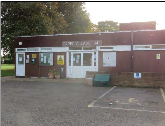
Capel Village Hall, located in Five Oak Green
