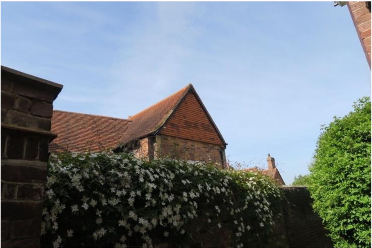
Figure 22: House showing typical tiled gable
