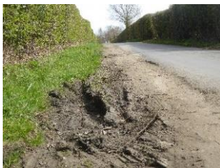
Eroded KCC Verge on A21 Rat Run lane (Spring 2021 in lockdown)_
