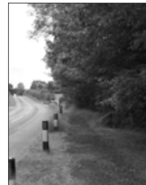
Concrete kerbs and plastic bollards
