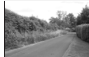
Cleared ditch with bund from arisings, now covered with vegetation
