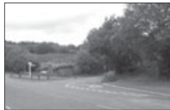
Restored narrowed junction
