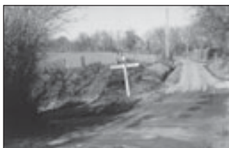
Awkward junction in narrow lane
