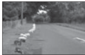
Painted concrete markers
