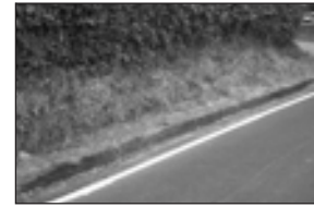
Timber sleeper kerbing
