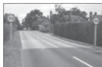
Applied aggregate to junction
