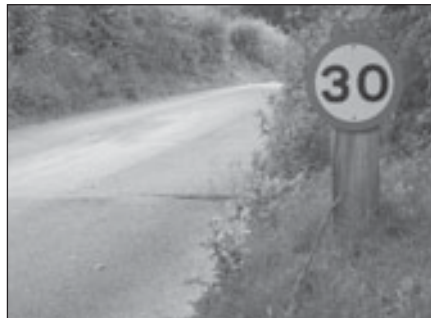
Example of small signs on short posts
