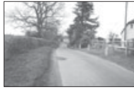
Timber bollards with timberpost and rail fence
