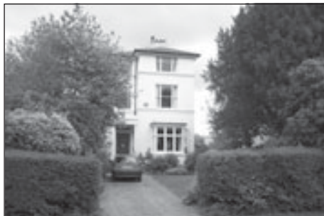
No 20 Park Road typifies the area
