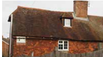
Half-hipped roof & clay tile hanging
