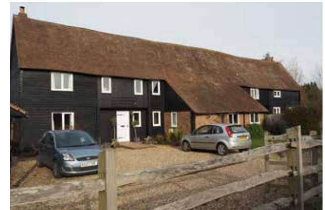
Figure 141: Weatherboarding or half weatherboarding and half red brick is a common technique used in the rural settlements in the parish and thus, new development should replicate this style to create a sensitive design outcome that respects the surroundings.
