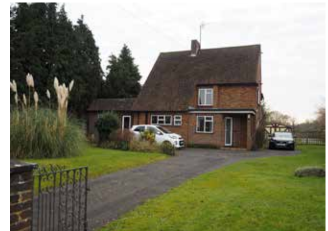
Figure 67: Local example of on-plot side parking and on-plot front parking with vegetation to provide screening. These parking solutions avoid cluttering the front façade of the house.
