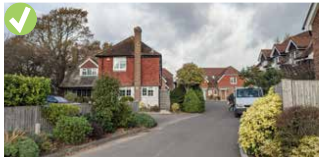
Figure 136: Positive example of small scale development within a rural village elsewhere in UK that respects the surrounding density, while also using the local vernacular as reference and integrating physical boundary treatments to create a pleasant visual outcome and a green buffer with surrounding existing properties.
