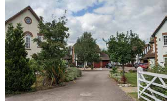
Figure 73: Example of a cul-de-sac street which includes only on-plot garage parking typologies, however, the strong presence of vegetation enhances the softness and rurality of the area mitigating any feeling of a car-dominated environment, elsewhere in UK.
