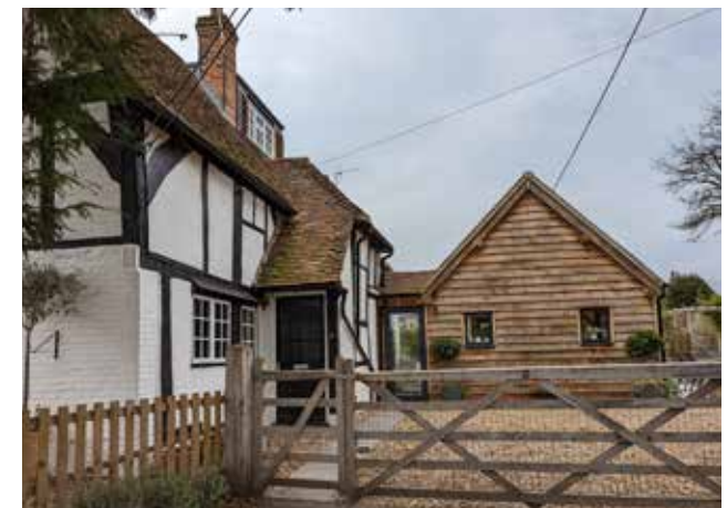
Figure 132: Positive example of a side extension that respects the existing building in terms of scale and building materials. In particular, the use of weatherboarding positively reflects back to the typical appearance of barns and outbuildings, elsewhere in rural UK.
