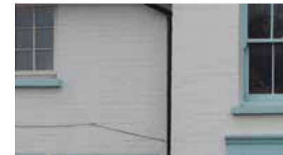
Off-white painted brickwork
