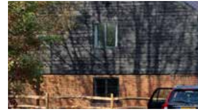
Half weatherboarding & half red brick
