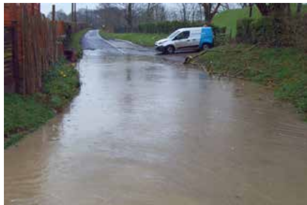
Figure 95: Flooding on Sherenden road.
