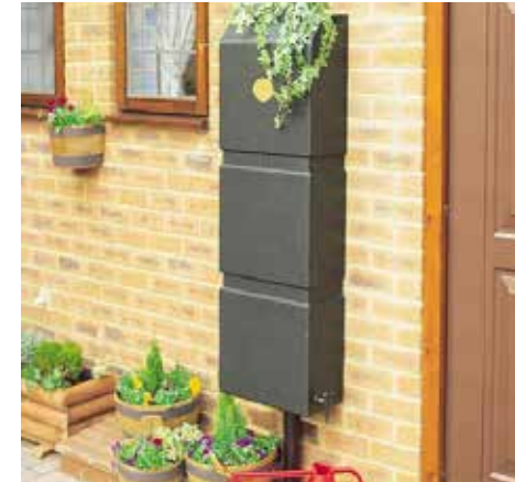
Figure 100: Example of a gravity fed rainwater system for flushing a downstairs toilet or for irrigation.
