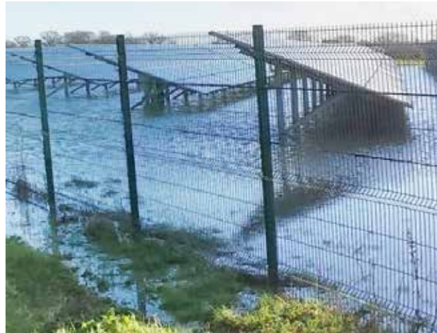
Figure 94: Flooding of the Solar Farm.
