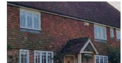
Clay tile hanging
