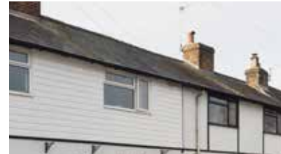
Pitched slate roof (continuous due to terraced typology)
