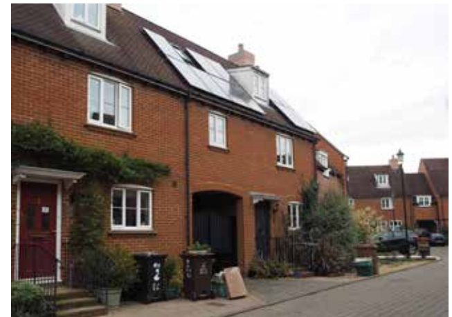
Figure 108: Local example in Ellis Close of implementing solar panels since the design stage.
