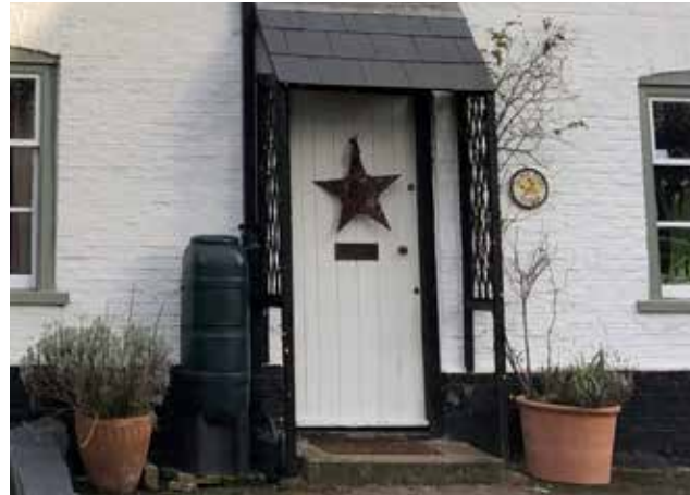
Figure 99: Examples of water butts used for rainwater harvesting in Reach, Cambridgeshire.
