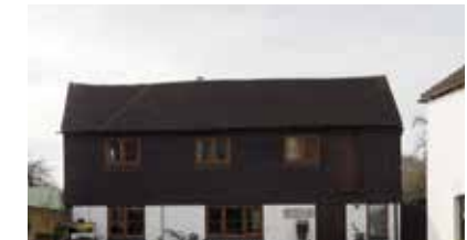
Black weatherboarding on first floor
