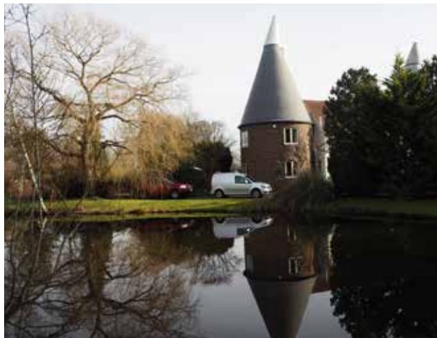
Figure 45: Local example of a short-distance view to the oast house, where the small pond acts as focal point around it, Whetsted.
