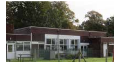
Flat roof (community building)
