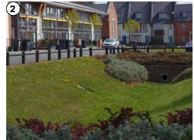
Figure 81: Green space overlooked by properties improving the environment, whilst also acting as a SuDS corridor.
