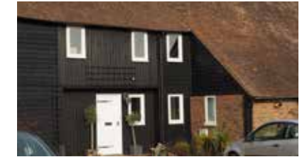
Black weatherboarding & cat slide roof
