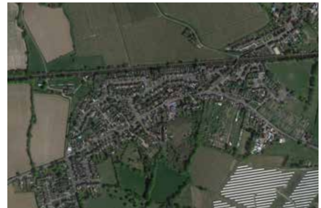
Figure 124: Example of a higher density settlement (approx. 35-40 dph) with reduced gaps between properties, whilst the size of rear gardens is smaller, Five Oak Green village. Any new development in close proximity needs to reflect the surrounding density, whilst go lower on the edges to allow for smooth transition to the countryside.
