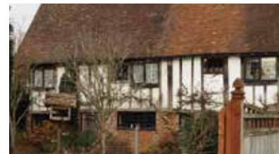
Timber frames with render infills
