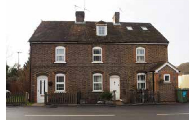
Figure 130: Local example of front extension to a building in Five Oak Green.
