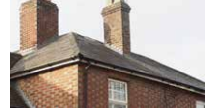
Hipped roof and blue brick header detailing
