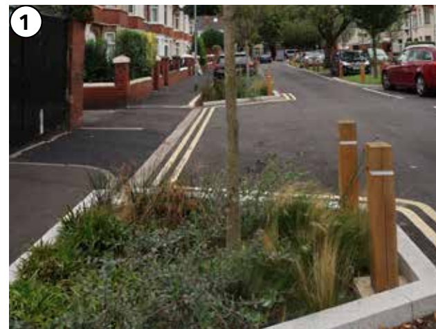
Figure 82: Example of a bioretention tree along a residential street. Those trees could also be retrofitted into existing roads.
