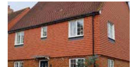
Modern example of tile hanging (concrete tiles)
