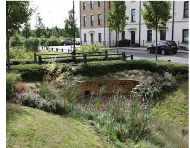
Figure 97: Example of swales check dam integrated with a crossing point, somewhere in UK.
