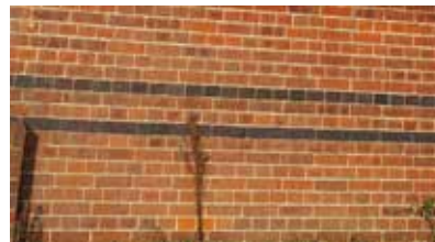
Red light multi brick with blue brick banding
