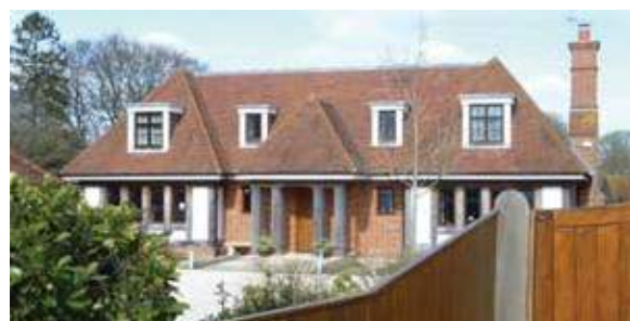
Rooms in roof with lower ridge — clay tiles
