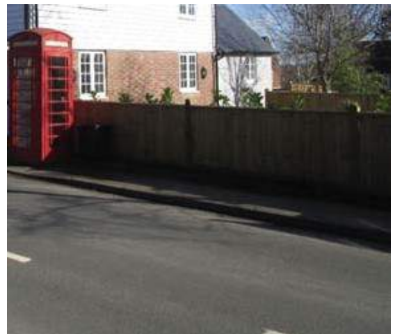
Medium-height close-boarded fence with timber posts
