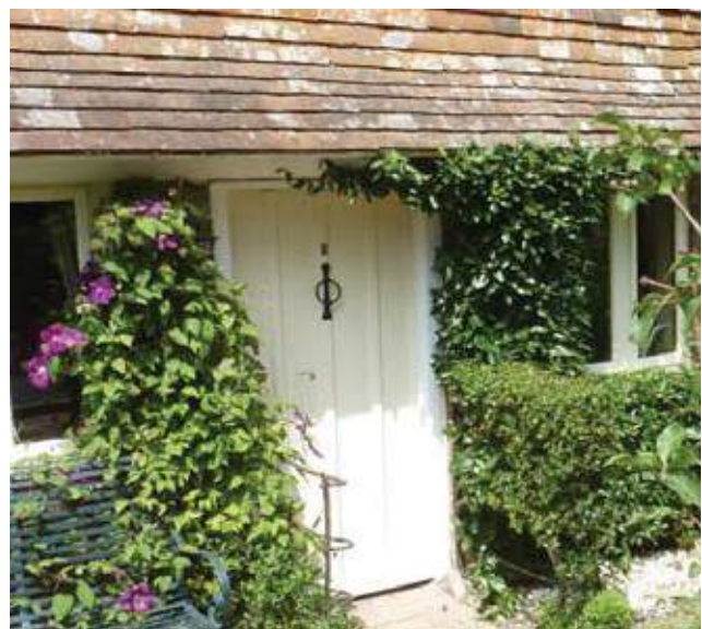
Canopy formed as roof over, with hanging tiles
