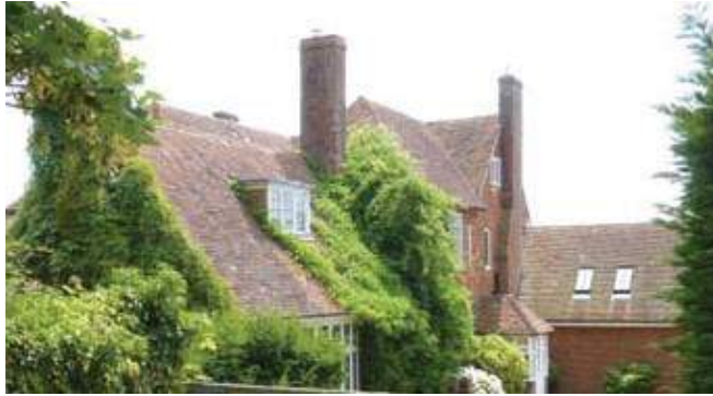
Different roof levels — Kent peg tiles
