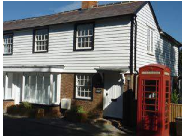
Weatherboarding above ground floor level
