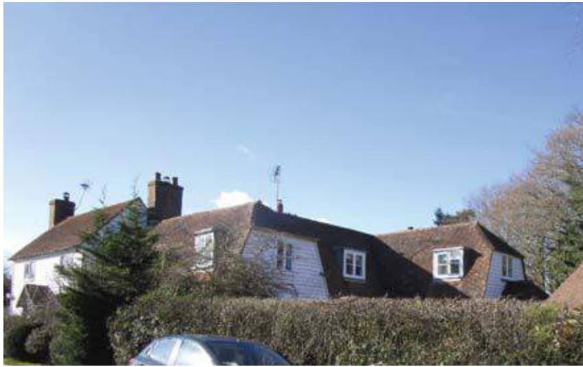
Rooms in roof with lower ridge — Kent peg tiles
