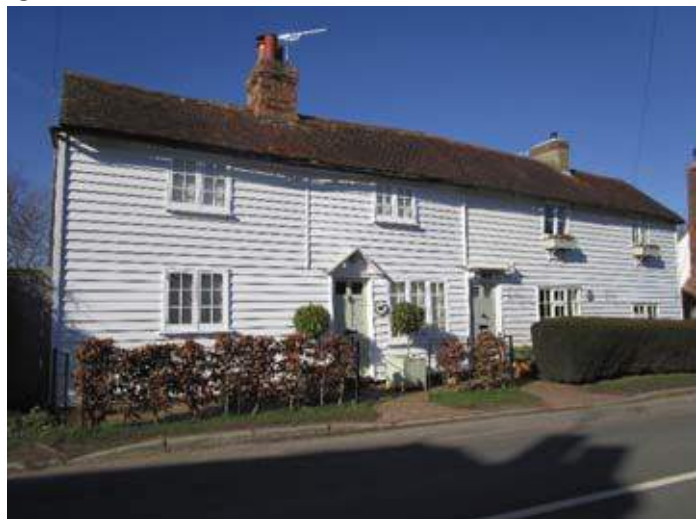
Simple roof structures with gable ends — Kent peg tiles
