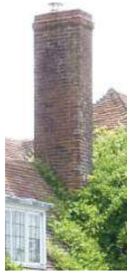
Tall chimney, exhaust above high ridge level
