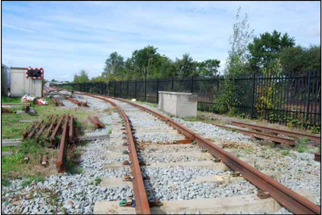
Plate 15: Portion of probably modern tracks along original PWH BL within Network Rail training facility, looking west.
