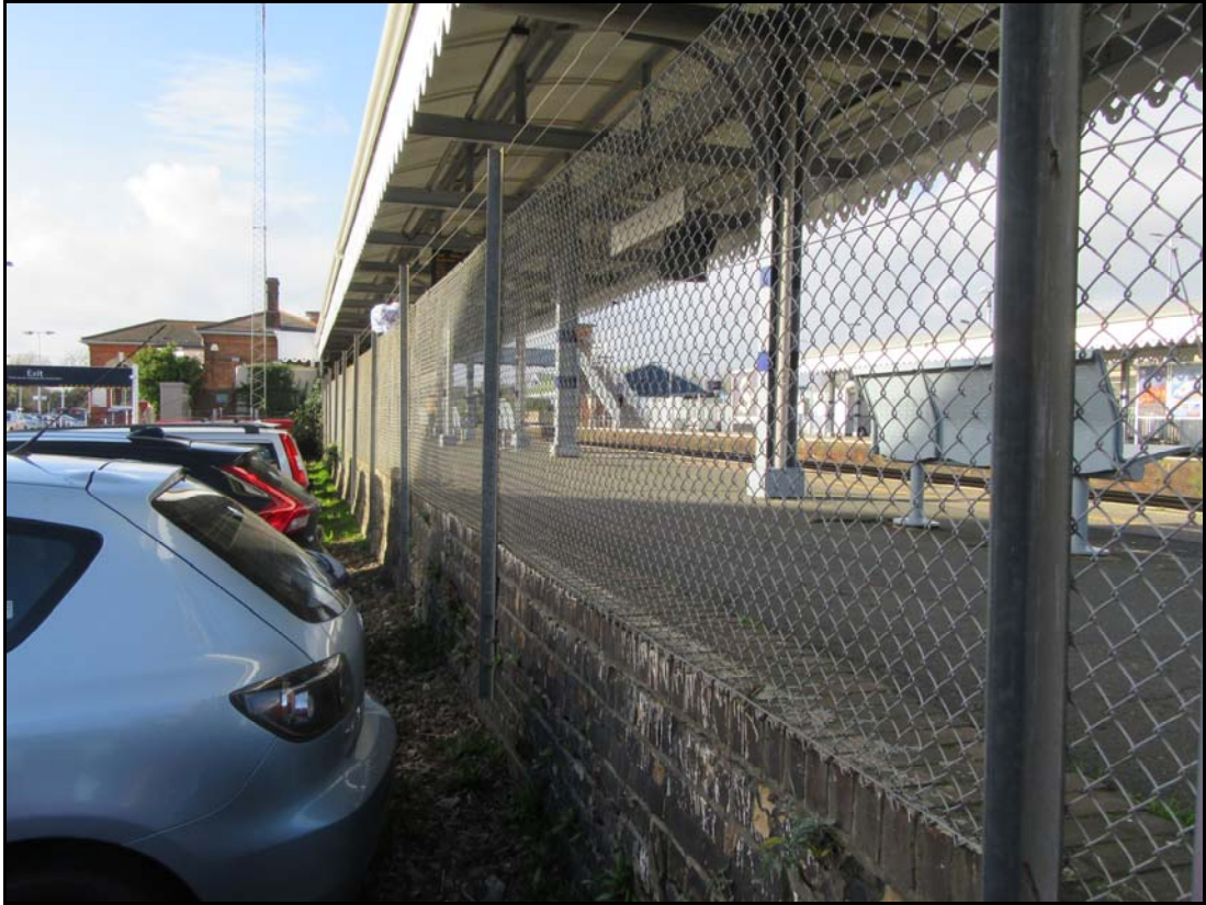
Plate 13: Southern side of platform serving the PWH BL which is still extant today (Image courtesy of D Sargison).
