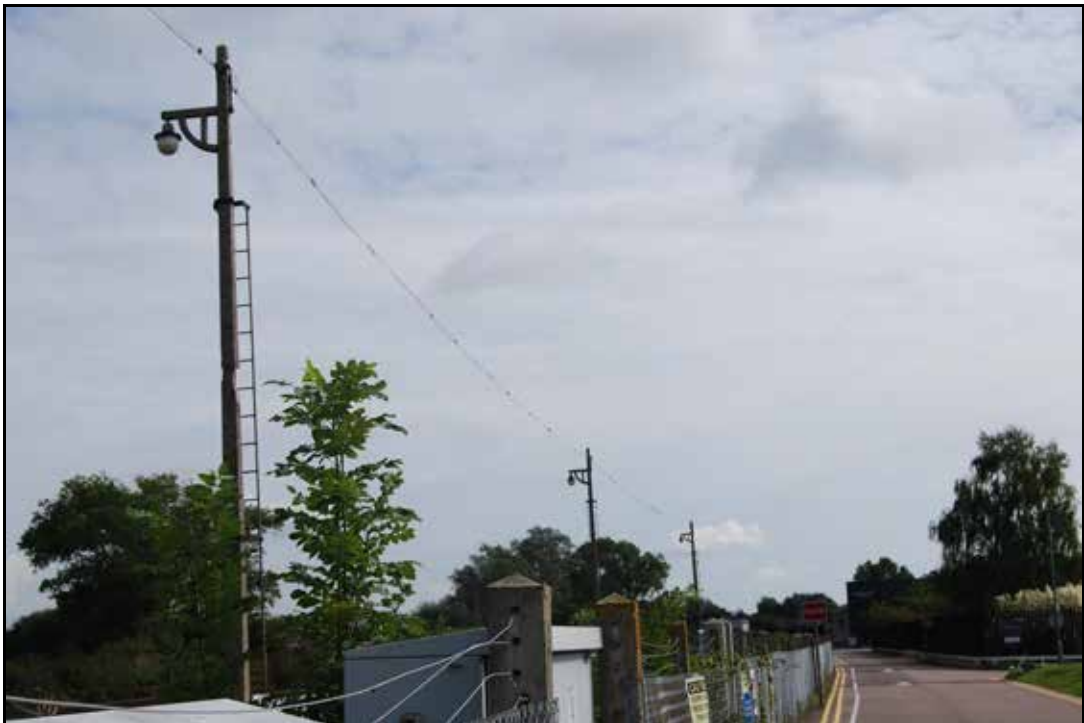
Plate 14: Lamp posts along road to east of Paddock Wood Station leading to Network Rail training facility.
