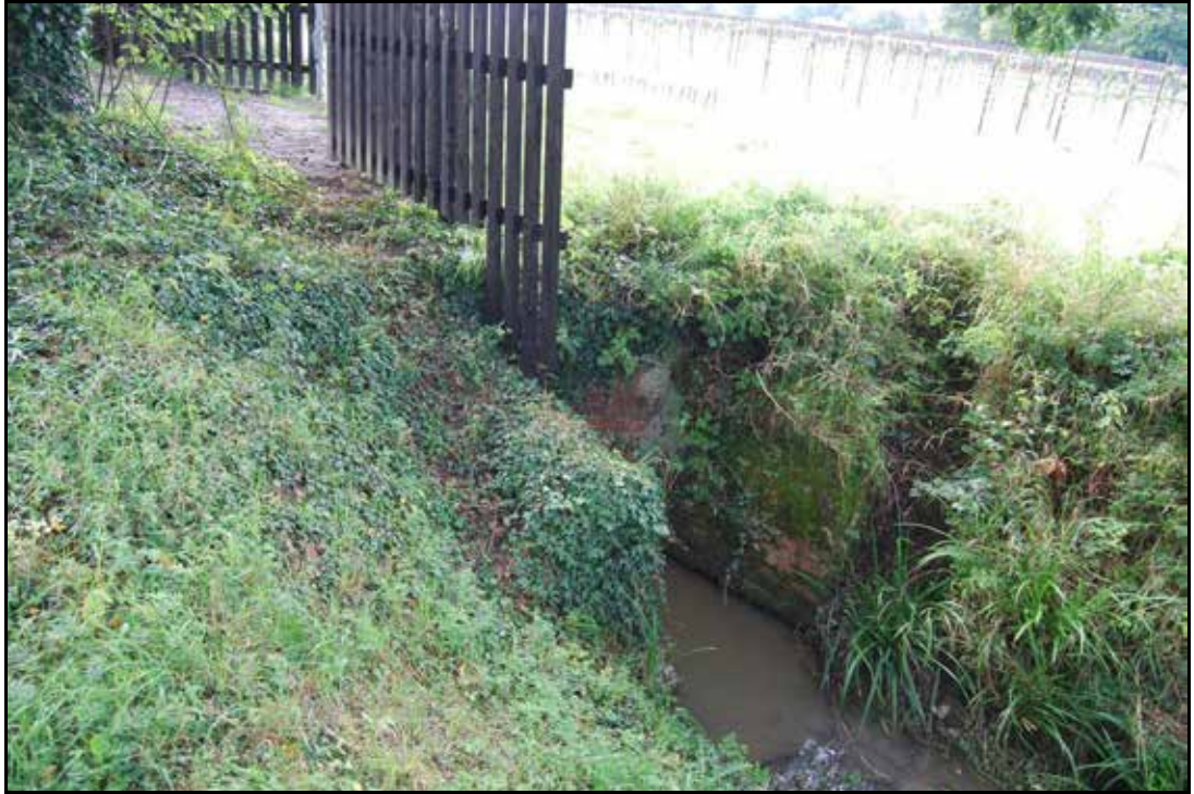
Plate 19: Brick bridge or culvert over stream on Willow Lane.
