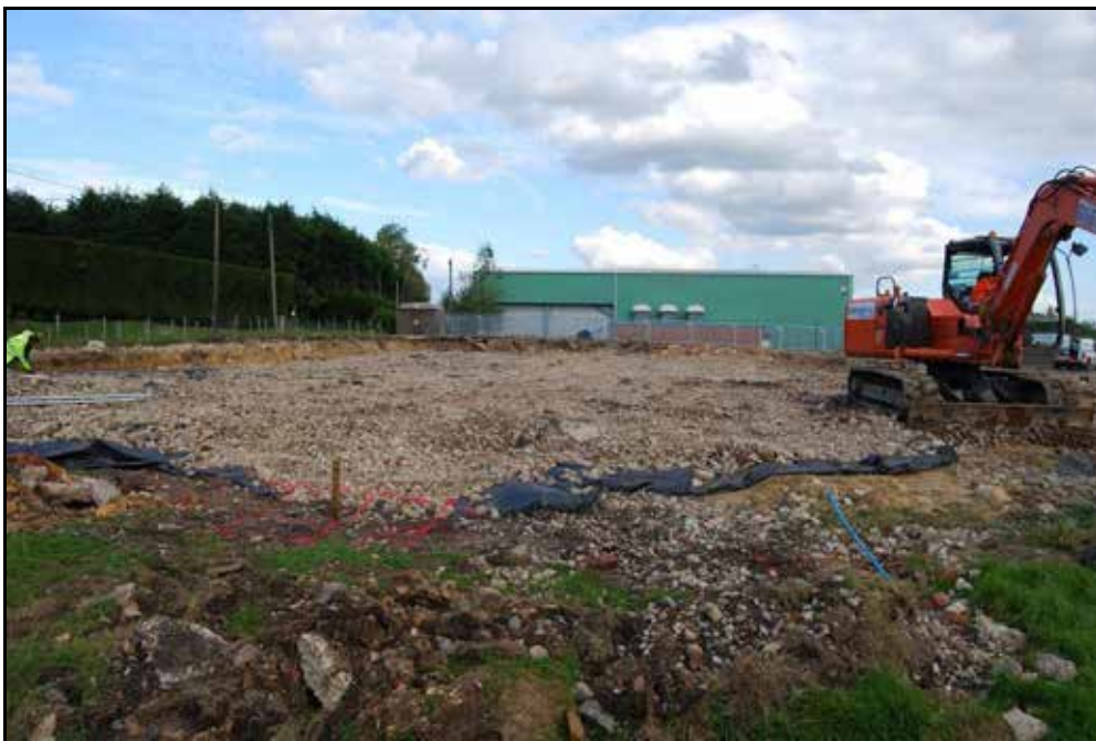
Plate 49: Current building site within former Hawkhurst Station area. No PWH BL remains were noted during site walkover.
