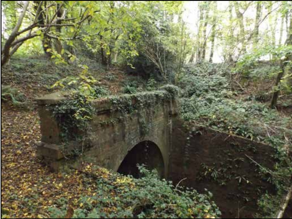
Plate 40: Surviving brickwork crowning tunnel entrance at Badgers Oak.
