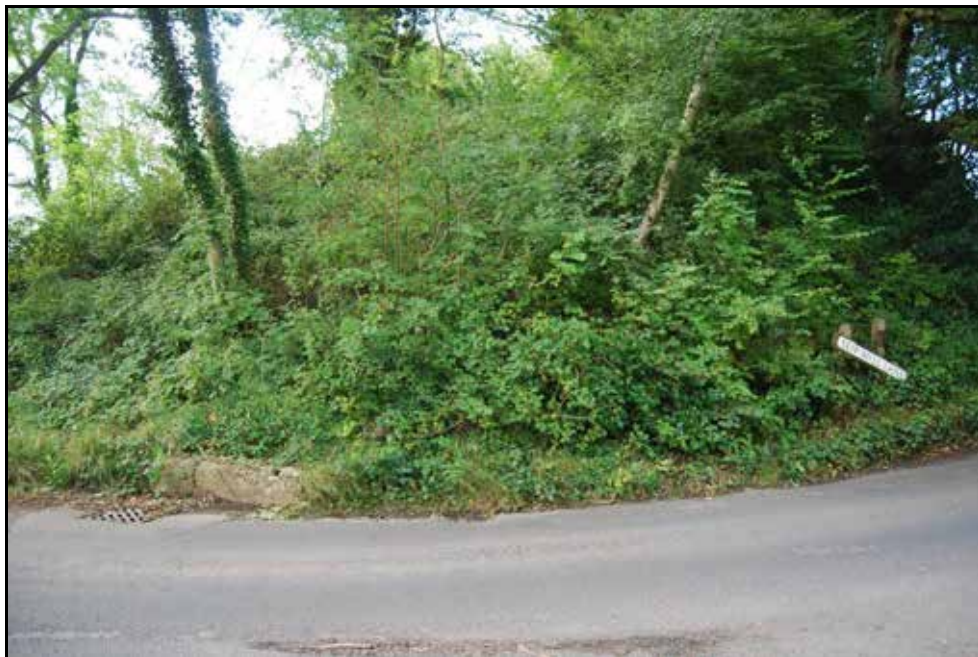
Plate 41: Part of PWH BL railway embankment adjacent to Slip Mill Road looking north.
