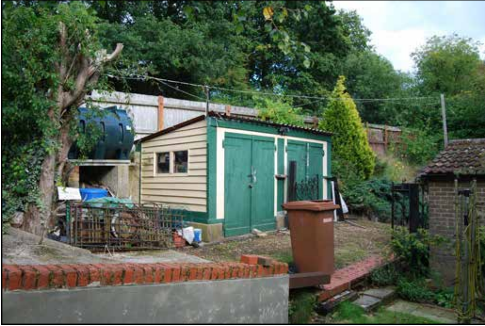
Plate 32: Shed and former platform edging bricks in garden at Cranbrook Station.
