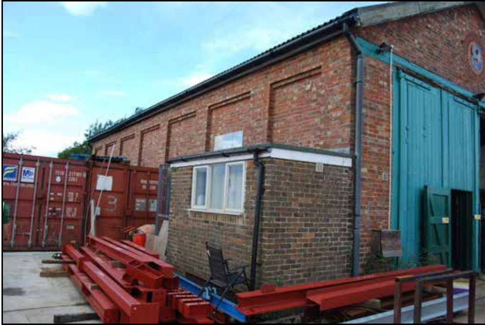
Plate 48: South western façade of engine shed with considerable amount of modern obstructions.
