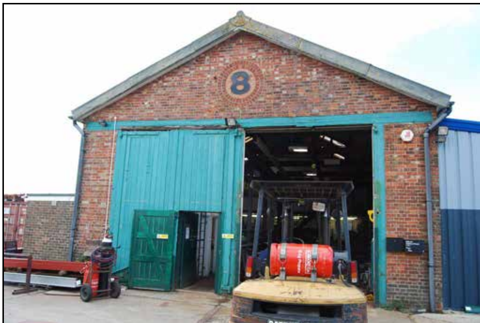
Plate 45: Front of the engine shed at Hawkhurst Station.
