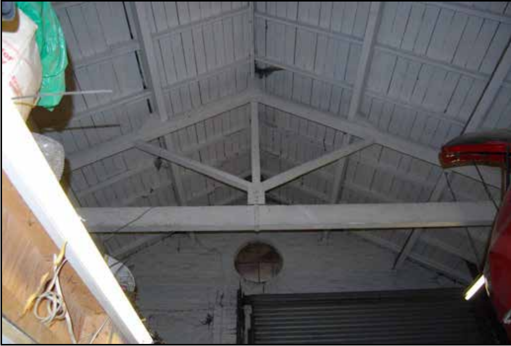
Plate 36: Internal joists, fixtures, fittings and circular window at Cranbrook goods shed.
