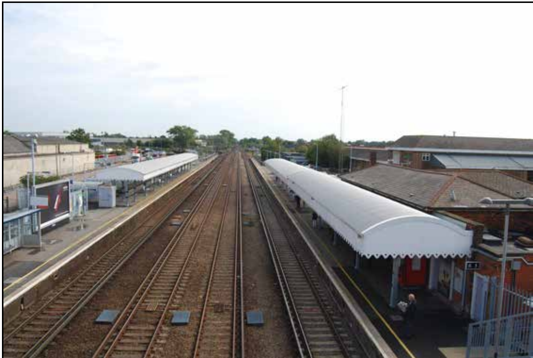
Plate 12: Paddock Wood Station down lines towards Maidstone, viewed from foot bridge looking east.
