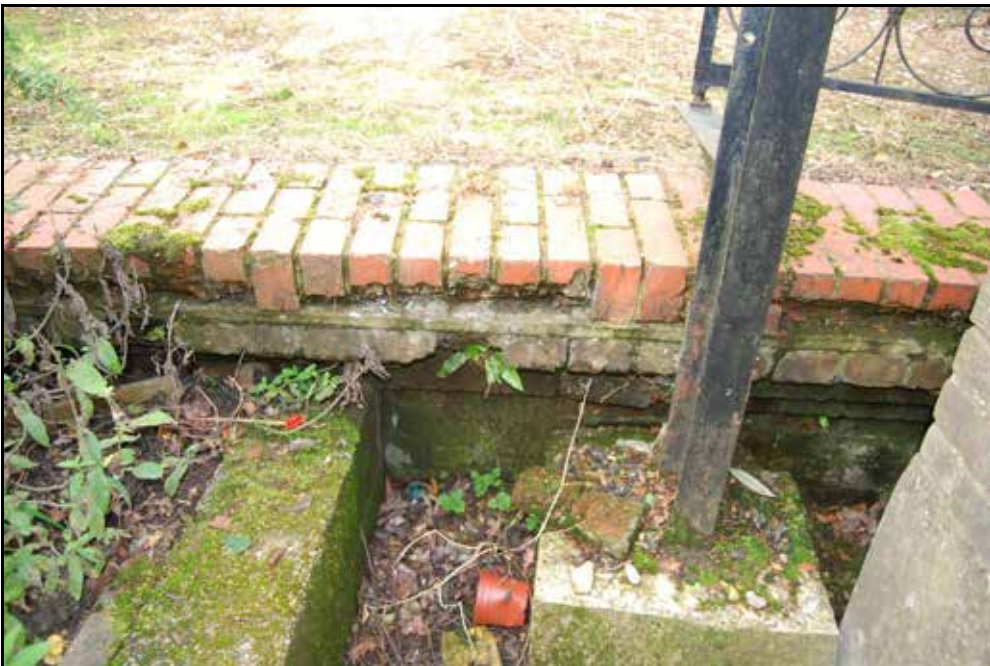
Plate 33: Close-up of brickwork of former platform at Cranbrook Station.
