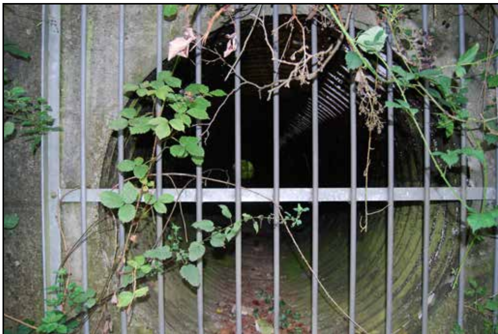
Plate 29: Culvert, which presumably replaced tunnel, running underneath Bedgebury Road, looking west.
