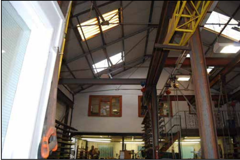
Plate 46: Internal detail and modern alterations (such as mezzanine floor) within former engine shed.
