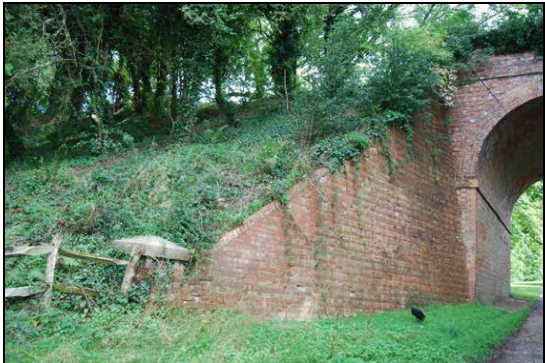
Plate 24: View of northern side of railway arch and embankment at Swigs Hall.
