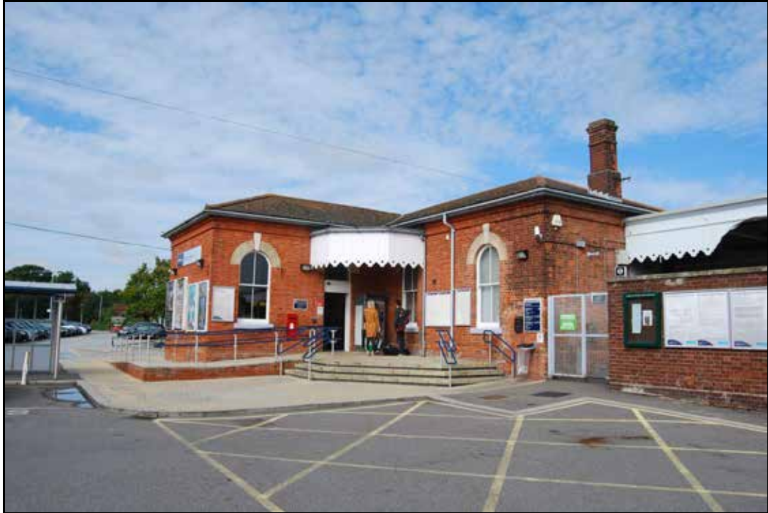
Plate 11: Front of Paddock Wood Station from approach road.
