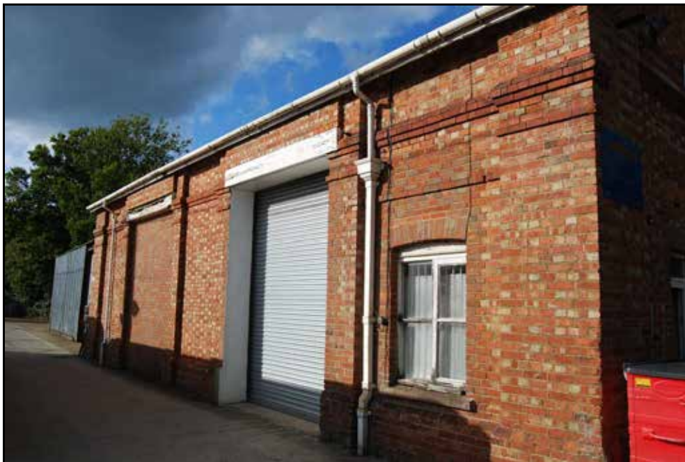
Plate 37: External façade of goods shed at Cranbrook Station.
