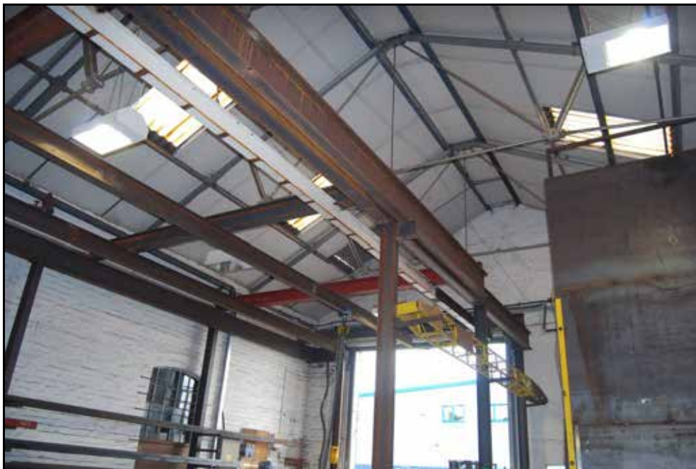
Plate 47: Internal detail and bricked-up circular window of engine shed.
