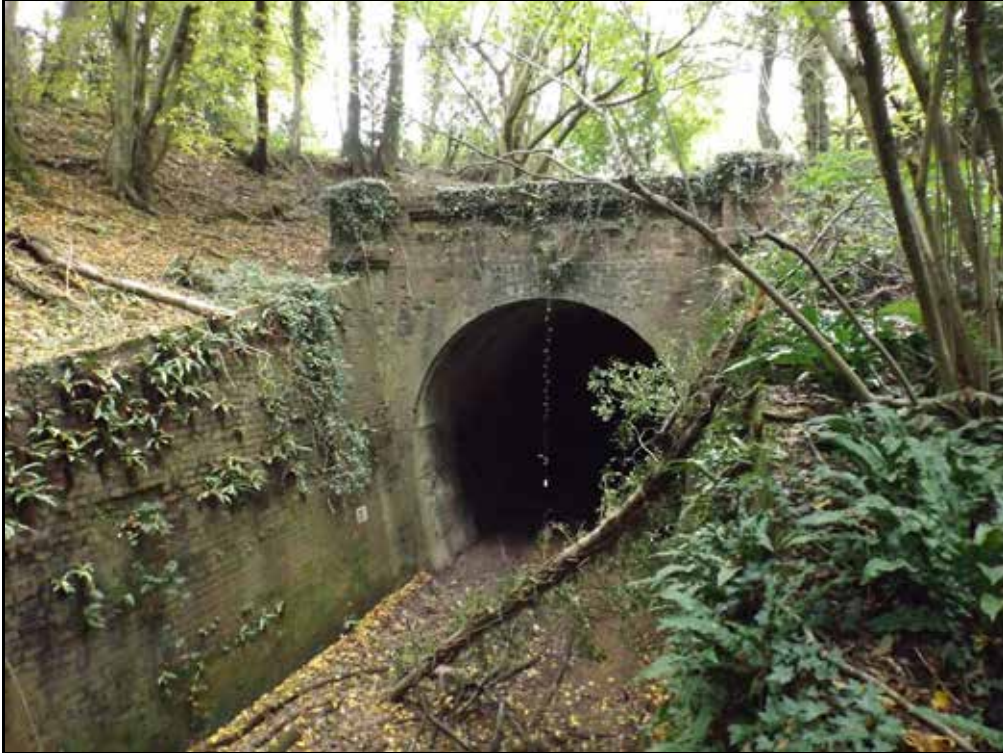
Plate 38: Entrance to Badgers Oak Tunnel, looking north.
